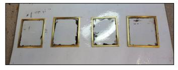
Once the window frames and glass had been cleaned, I sanded down the brass frame for a better bond, preparing them so that the long process of covering the outside edges with a wooden veneer could begin.
